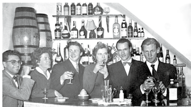
The bar at Calle San Fernando
